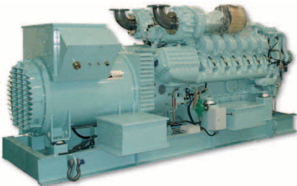
1350 kW emergency generating set with MTU diesel engine
